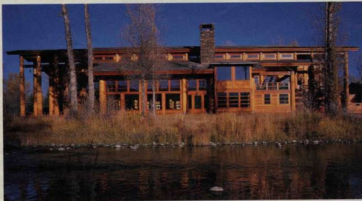
Rural Sprawl Glass and wood panels are set into a frame defined by log columns, with low-pitched roofs extending beyond the main structure.
